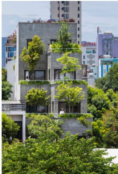
Hình 6.2.5: Green Peace Village Đà Nẵng | Green Peace Village, Danang Source: Ho Khue Architects
