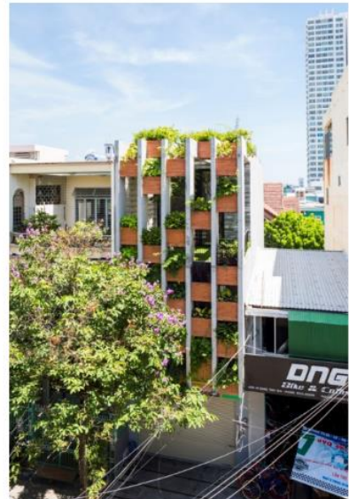
Hình 6.2.6: Resort in House, Đà Nẵng | Resort in House, Danang Source: Hiroyuki Oki
